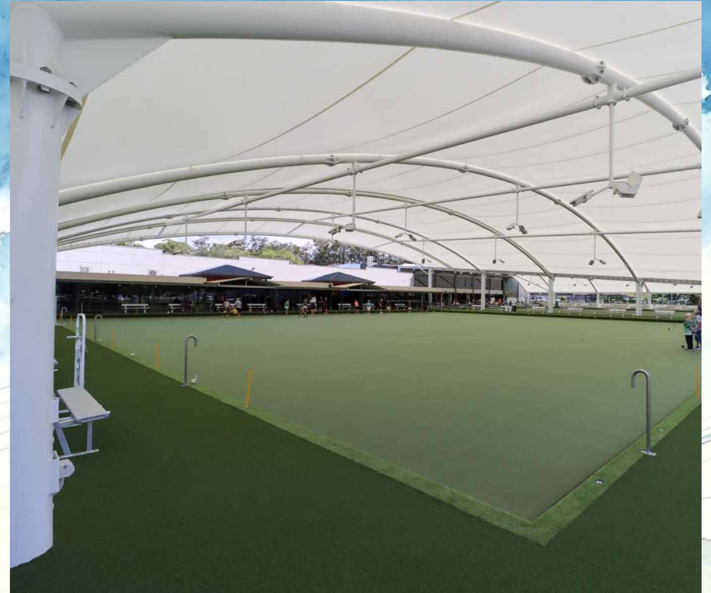
草地滚球俱乐部顶棚 · Bowling Green Tensile Roof
