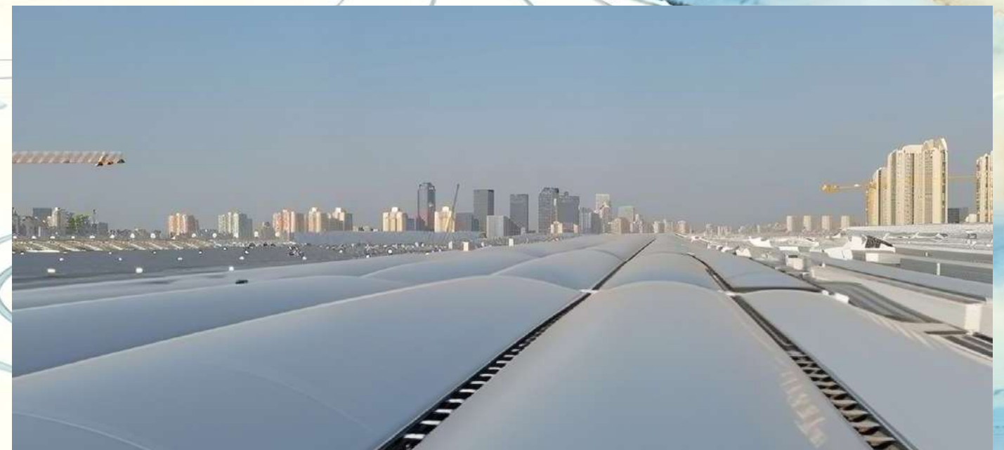
北京丰台站 · 中央光庭ETFE膜结构 · Beijing Fengtai Railway Station - Central Atrium ETFE Membrane Structure
