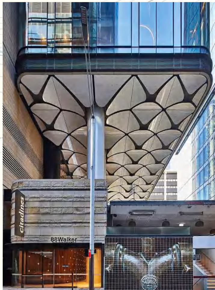
沃克街88号建筑下表面 · 88 Walker Street (North Sydney) - Cantilever Soffit / Underside
