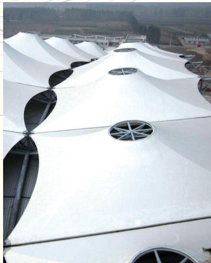
河北唐山机场 · Tangshan Sannvhe Airport Terminal Membrane Structure Roof
