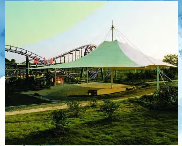
江苏宜兴森林公园 · Yixing Longbeishan Forest Park Roller Coaster - Membrane Structure Canopy
