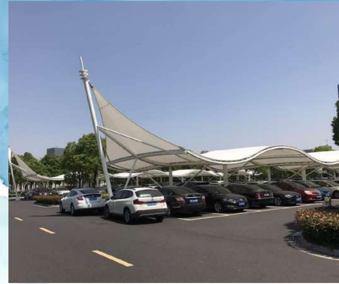
吴江停车场 · Wujiang Membrane Structure Parking Lot/Canopy
